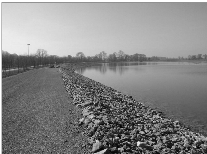
Figure 8.1 Typical bank protection (courtesy Environment Agency UK)
