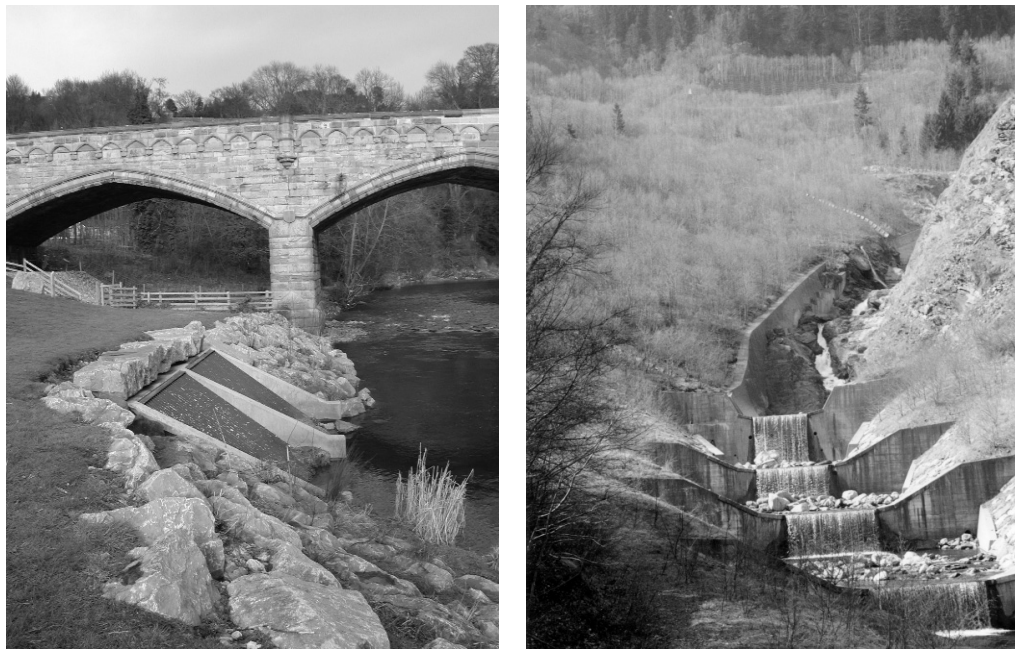
Figure 8.43 Example of armourstone used in a small river: (left) rock revetment used to protect a storm drain outfall structure on an upland river in Richmond (UK) (courtesy C Rickard) and (right) control of torrent in the vicinity of Felkskanal (Austria) (courtesy I Lotherat)
