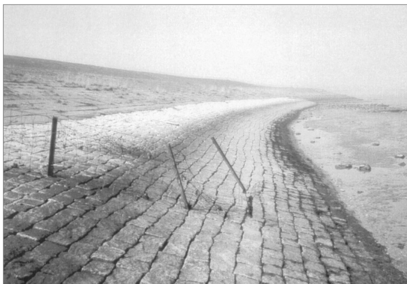
Figure 8.7 Revetment made of pitched stone (courtesy J van Duivendijk)
