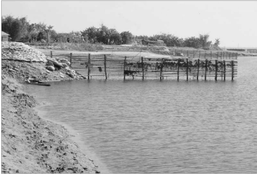
Figure 8.13 Hard points under construction (courtesy Witteveen+Bos)
