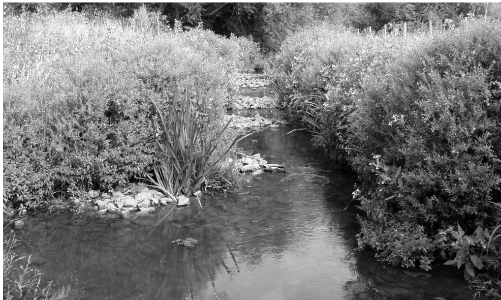
Figure 8.5 Rock structures in a small stream to stabilise the bed and create riffles (courtesy Mott MacDonald)
