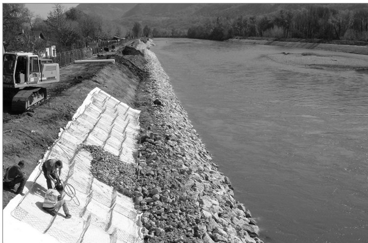
Figure 8.59 Construction of gabion revetments in wet or dry conditions (courtesy Maccaferri, France)
