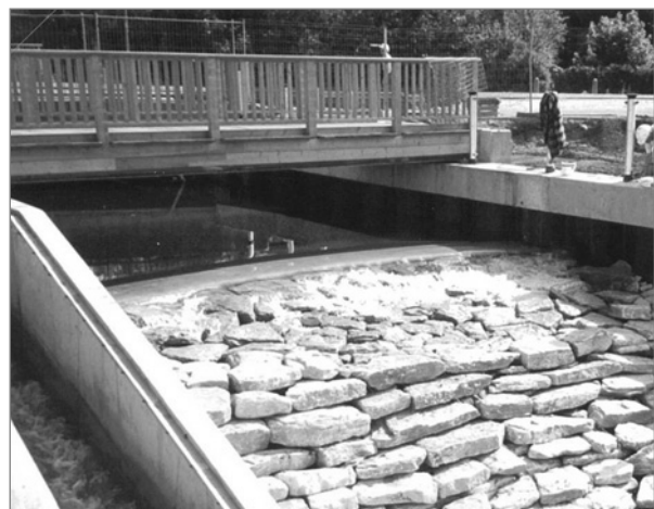
Figure 1.14 Seuil (source : A. Pepper)
