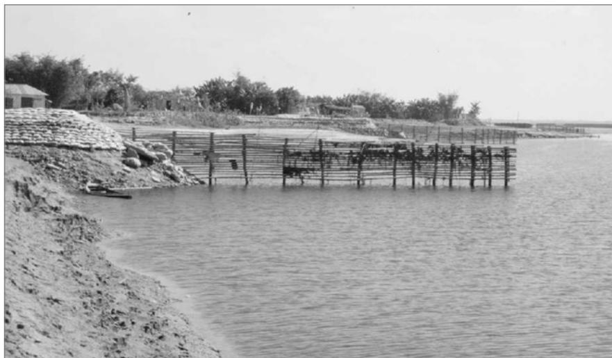
**Figure 8.13** Points durs en construction (source: Witteveen + Bos)
