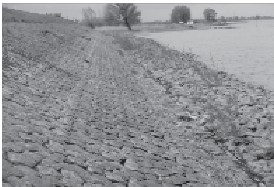
Figure 5.75 Toe (or SWL berm) of a river dike (courtesy Rijkswaterstaat)
