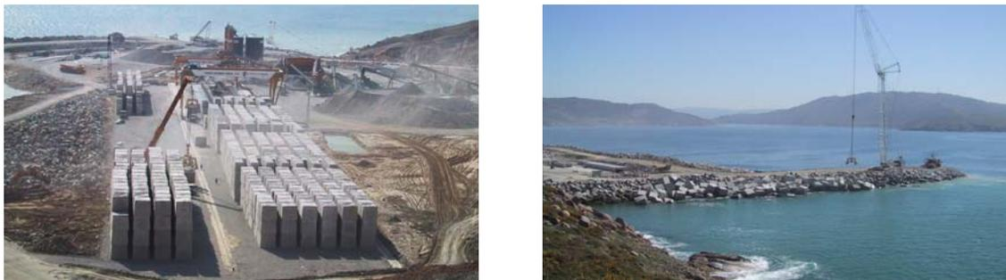
Figure 19. Block manufacturing yard and crane laying blocks.
