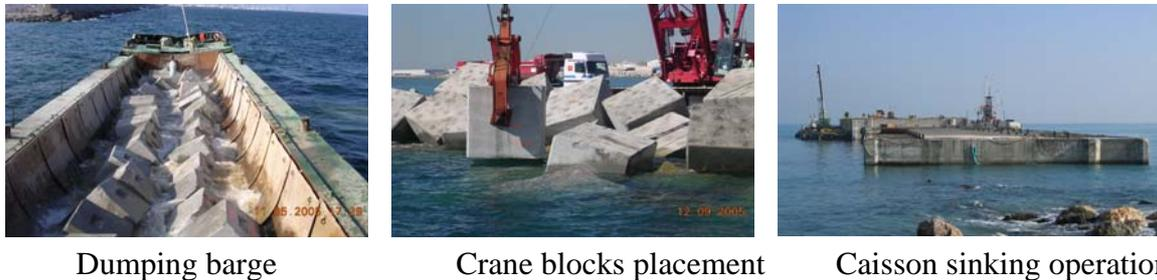
Figure 40. Breakwaters construction stages.
