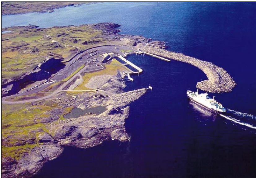
Mortavika Ferry Terminal, Norway Photo: Odd Furunes, Statens vegvesen
