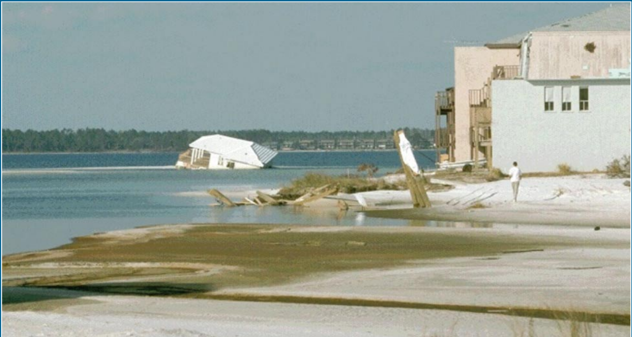
Possible consequences of coastline erosion Photo: From the Coastal Engineering Manual
