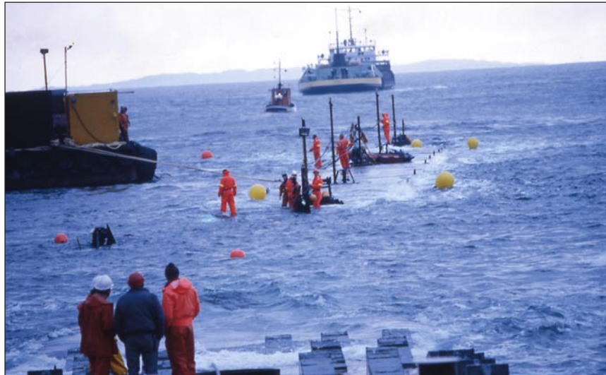
Pipeline landfall on western coast of Norway Photo: Ingeniør F. Selmer A/S
