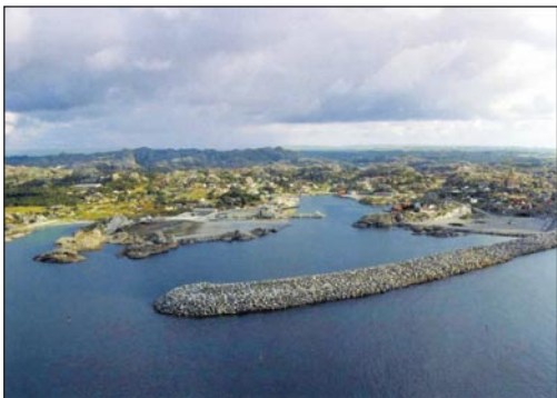
Sirevåg harbour Protection by berm breakwater Top: Laboratory model tests Middle: Numerical modelling Bottom: As built
