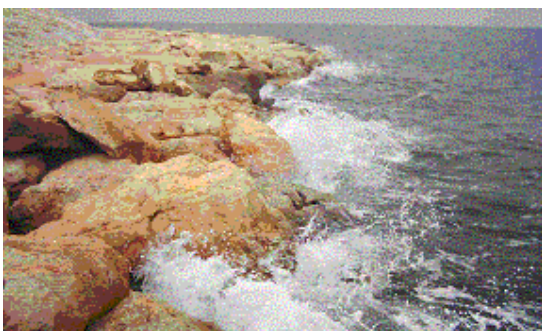
Fig 15 : Damage of edge in Berm
