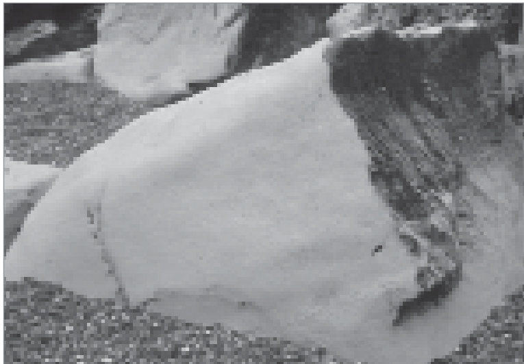
Figure 3.12 Rapid erosion and mass loss of oolitic limestone armour stones by shingle wear (courtesy J-P Latham)
