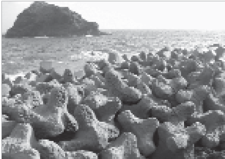
Figure 3.95 Example of Accropode and Ecopode used in combination (courtesy Sogreah)
