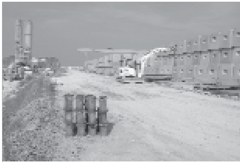
Figure 3.98 Example of units yard in Barcelona with dedicated high capacity handling frame. Note that units are casted alongside the yard and cylinder moulds for concrete quality control (courtesy S Dupray)
