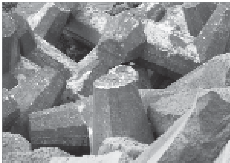
Figure 3.93 Example of Dolos used on slope with heavy basalt armourstone on crest (courtesy S Dupray)
