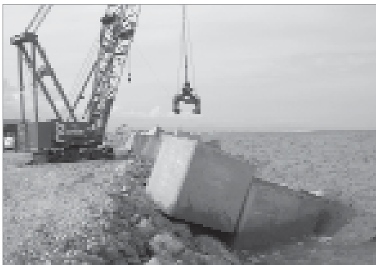
Figure 3.91 Example of cubic blocks being placed by cable crane during Barcelona breakwater construction (courtesy S Dupray)
