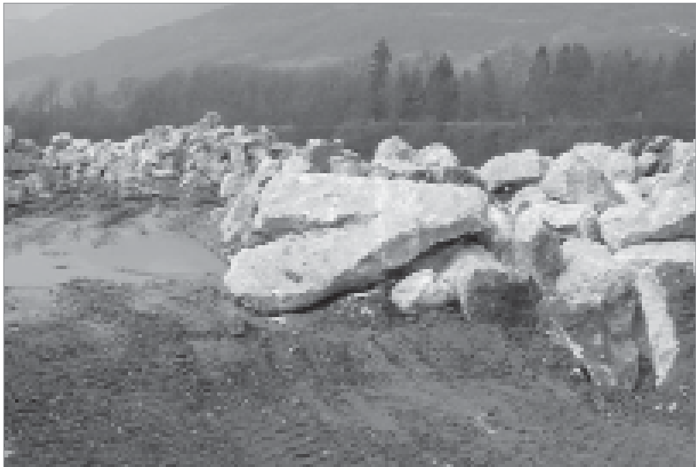
Figure 3.87 View of a temporary stockpile of 1000–3000 kg with inappropriate quality control (courtesy S Dupray). Stones with unsuitable shape and mass are in the deliveries. The different gradings are hardly separated and distinguished on site
