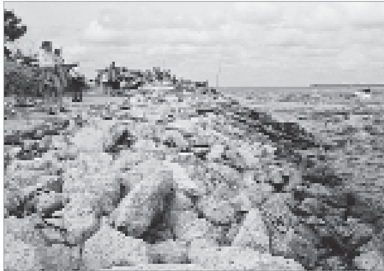
Figure 3.99 Example of the use of crushed concrete in a dike
