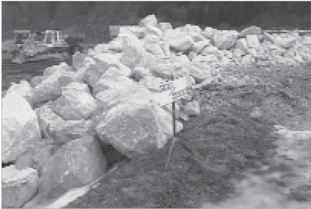
Figure 3.86 View of a temporary stockpile of 800–2000 kg where contamination by fine material and soil is visible (courtesy S Dupray). The board in the front clearly indicates the grading, which allows drivers to deliver to the appropriate stockpile
