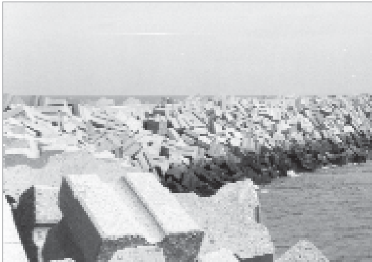
Figure 3.92 Example of Antifer cubes – Antifer breakwater (courtesy S Dupray)
