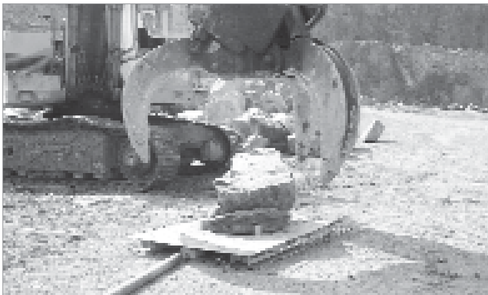
Figure 3.41 View of high capacity weighing scale made of portable weigh beams, used for blocks with a mass of less than 6 tonnes (courtesy S Dupray)
