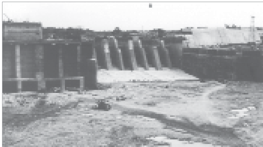
Figure 7.17 Diversion stage II of the River Niger at Kainji Dam will take place through unfinished spillway structures (courtesy J van Duivendijk)
