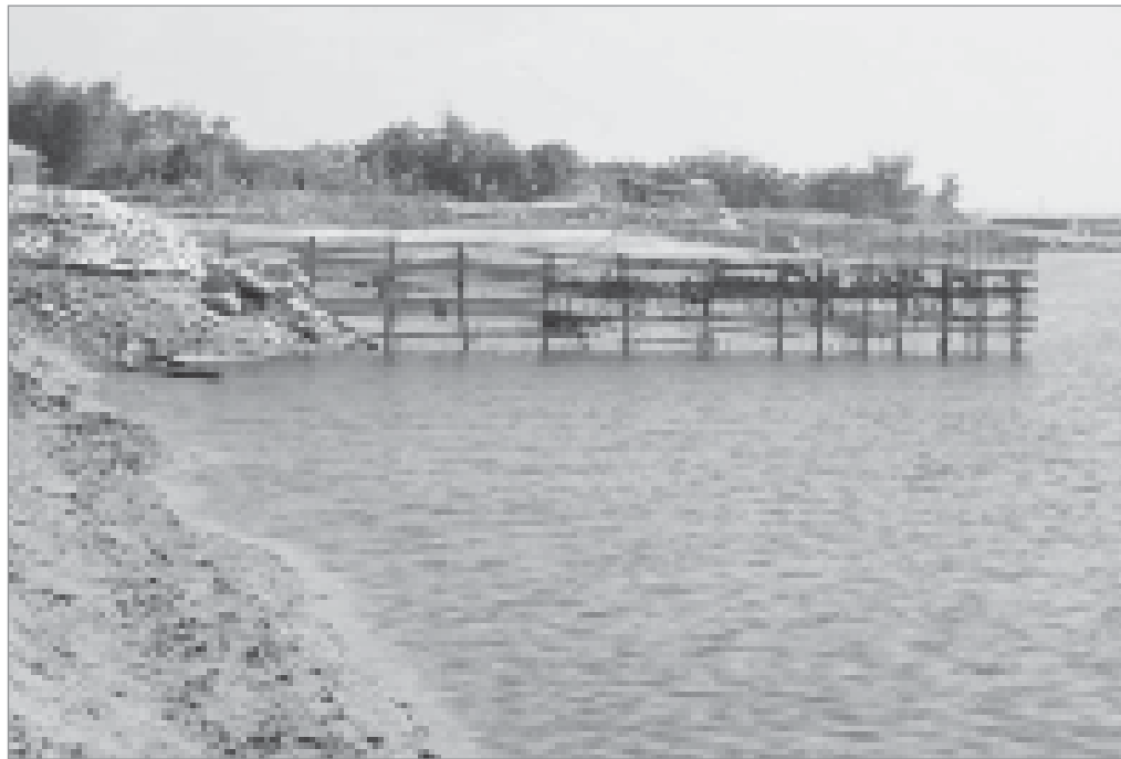
Figure 8.13 Hard points under construction (courtesy Witteveen+Bos)
