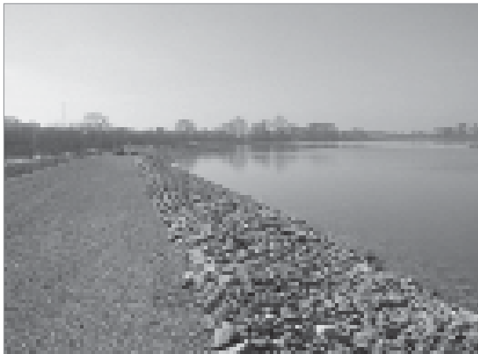
Figure 8.1 Typical bank protection (courtesy Environment Agency UK)
