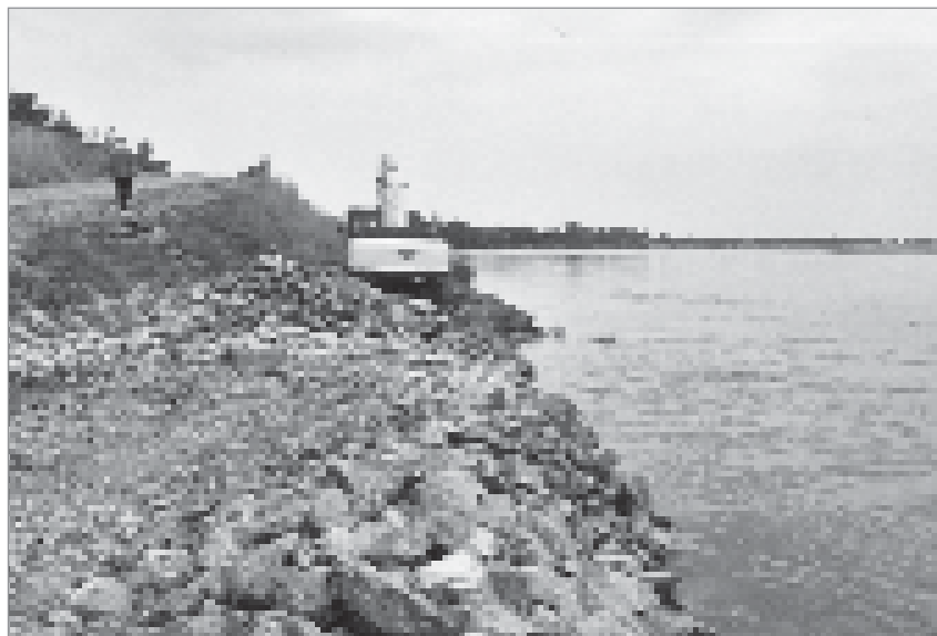
Figure 8.14 Flood protection dike along the Loire river under rehabilitation, notably the scour protection (courtesy TPPL France)
