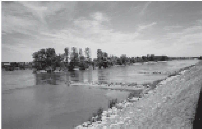
Figure 8.11 A system of spur-dikes on the river Loire (France) (courtesy Service Maritime et de Navigation de Nantes)
