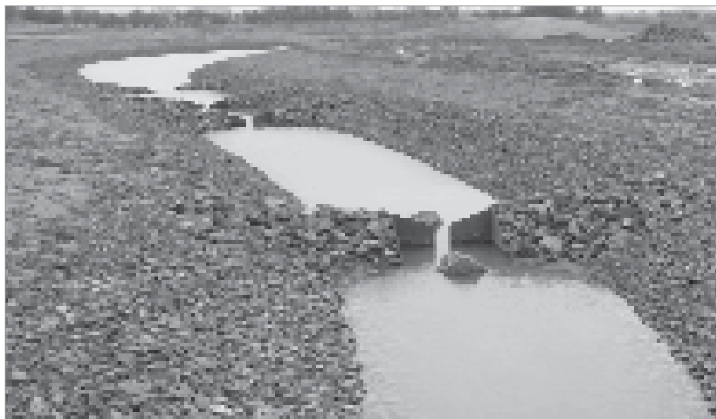
Figure 8.49 Fishway in the River Rhine showing V-shaped weir with vertical slot (courtesy Rijkswaterstaat)
