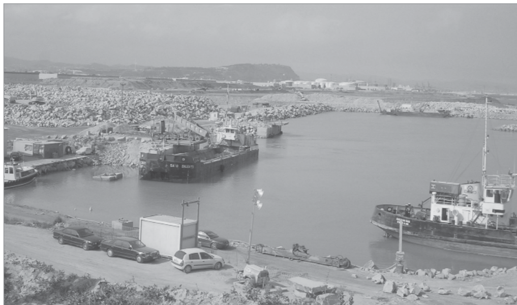
Figure 9.33 General view of Barcelona stockpile where trucks deliver stones to stocks or to a barge for onshore dumping (courtesy CETE de Lyon)
