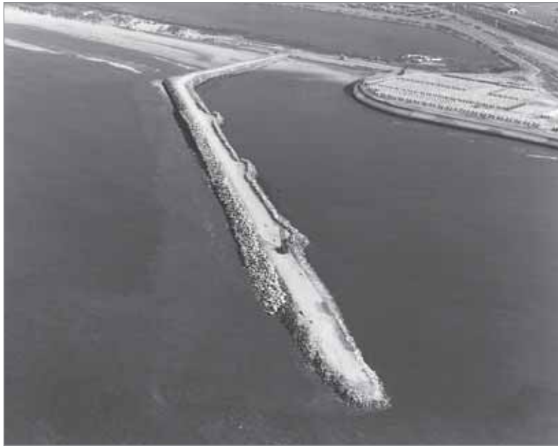
Figure 9.55 Placement of armour layer, showing expansions for turning and passing along the crest of the core (courtesy Van Oord)
