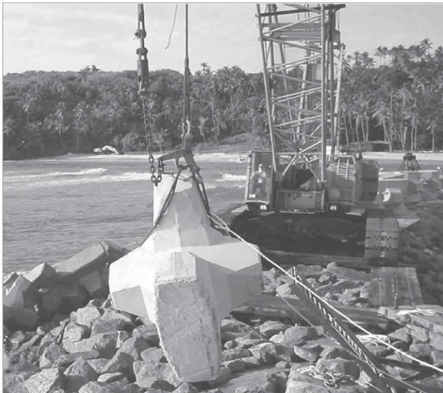
Figure 9.61 Use of a quick-release hook (courtesy Interbeton)
