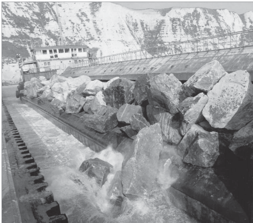
Figure 9.21 Side stone-dumping vessel Cetus dumping 1–3 t armourstone near a jetty (courtesy Royal Boskalis Westminster)
