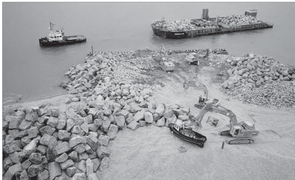
Figure 9.11 Unloading a sea transport barge (courtesy Royal Boskalis Westminster)
