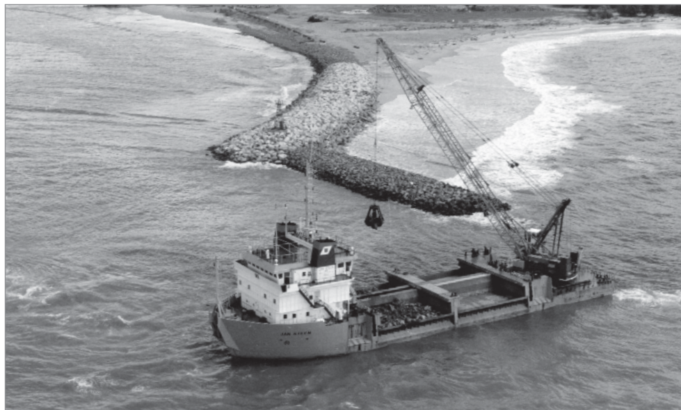
Figure 9.23 Crane mounted on the rock supply vessel Jan Steen (courtesy Van Oord)
