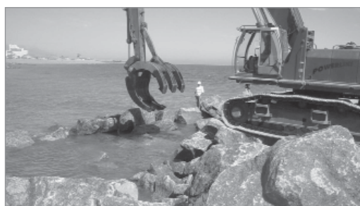
Figure 9.17 Examples of grabs used for armourstone placement (courtesy Royal Boskalis)
