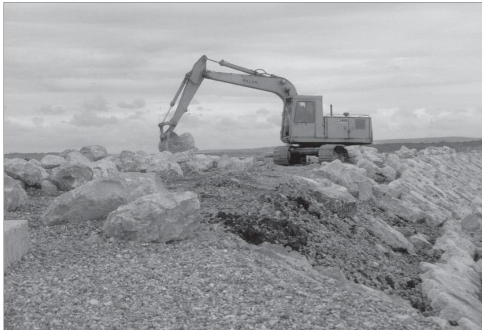
Figure 9.14 Excavator working on the crest (courtesy J D Simm)
